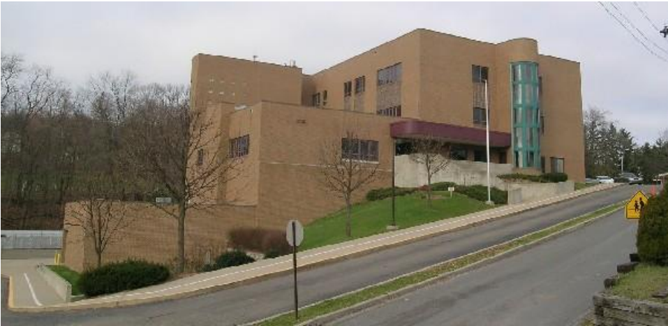
Claysville Elementary School
